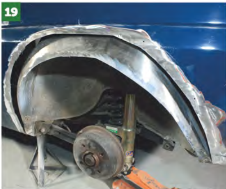
19 ...leaving the inner arch. That's if it's there, as it might be rusted and need replacement.
